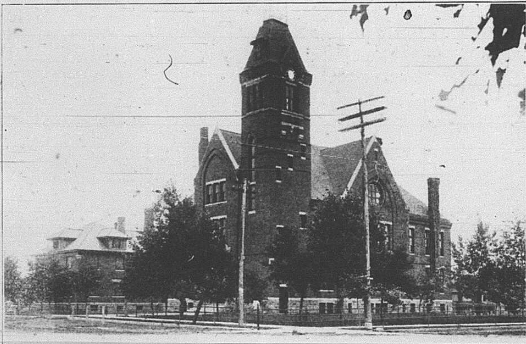
Stutsman County Court House, Located at Jamestown, North Dakota
