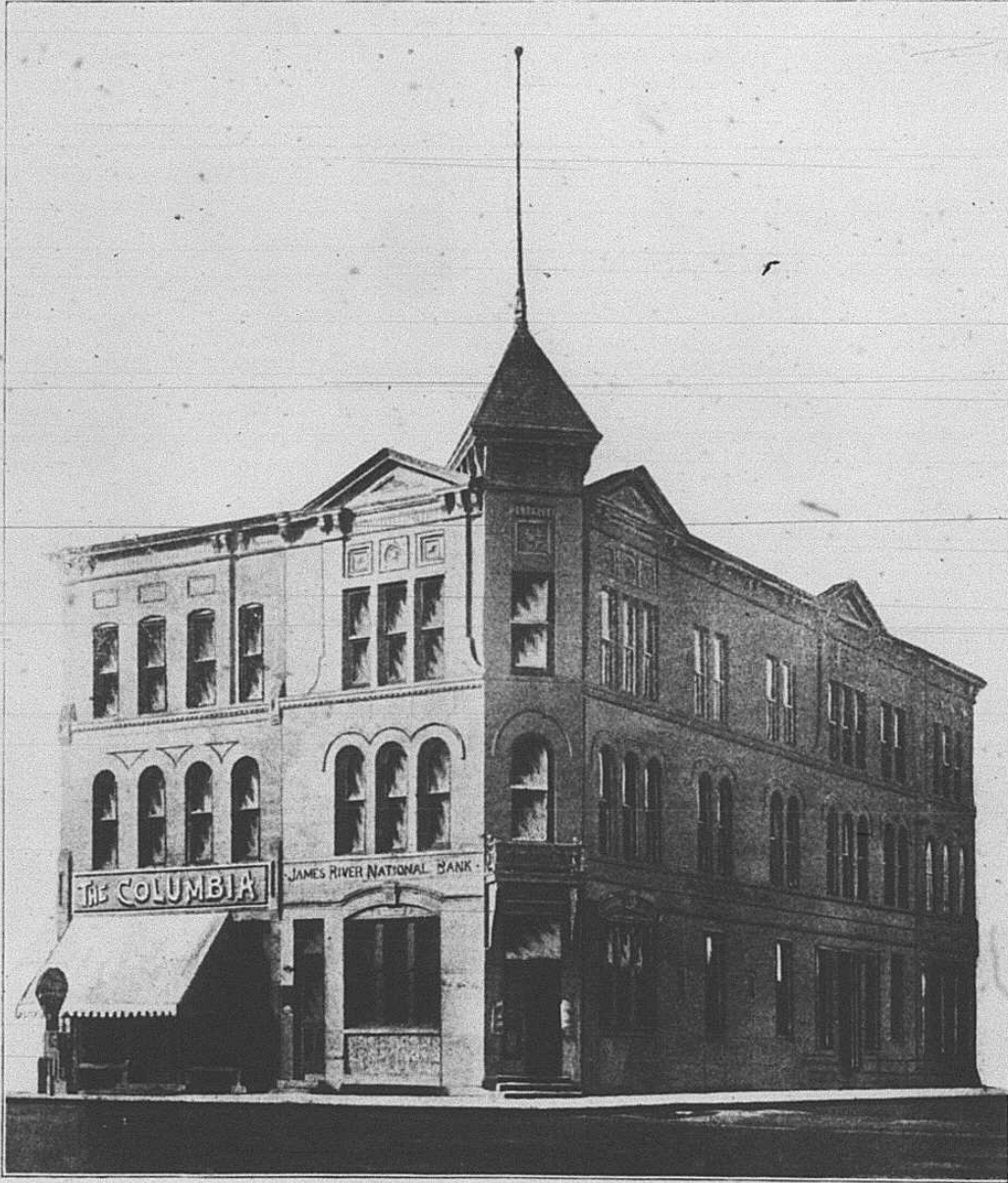
James River National Bank Building, Jamestown, North Dakota
