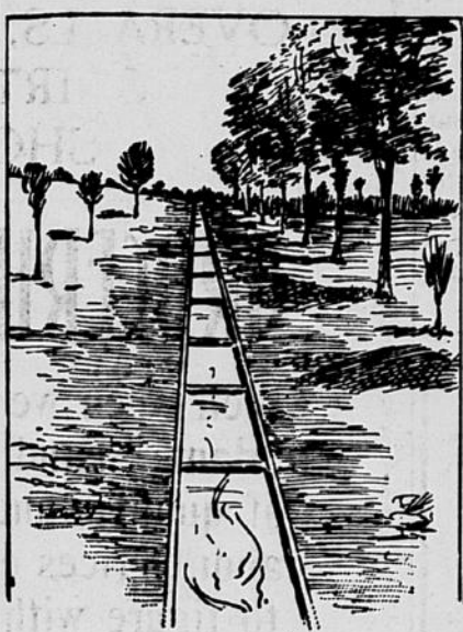
CONTINUOUS CEMENT FLUME.
