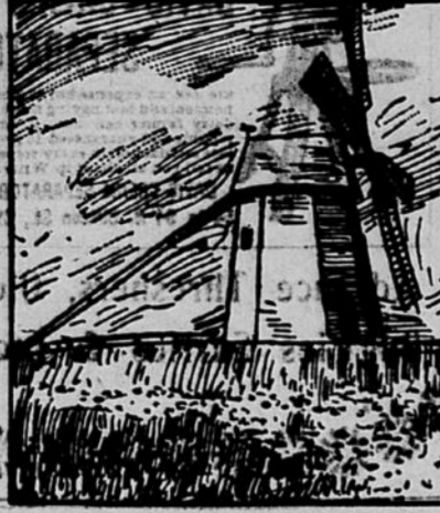
OLD CHATHAM WINDMILL. (It Was Built in 1797 and Still is Used for Grinding Grain.)
