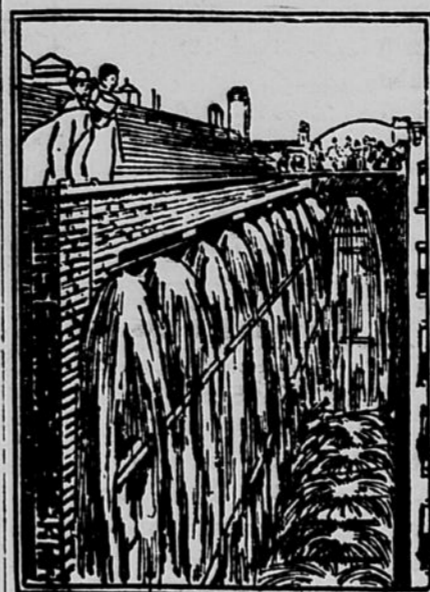
THE FIRE CURTAIN. (Showing Method of Operation to Prevent the Spread of Big Fires.)
