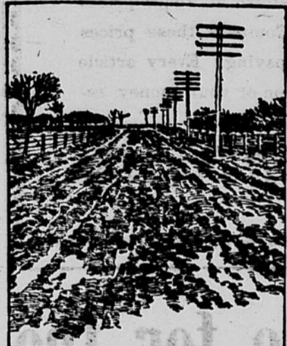
ROAD BEFORE IMPROVEMENT.
