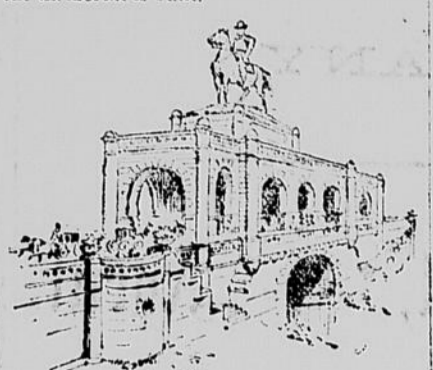
VIEW SHOWING ELEVATED ROADWAY.
