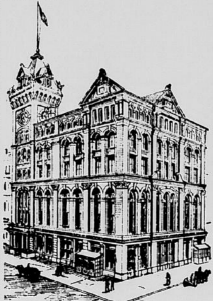
THE EXCHANGE BUILDING.
