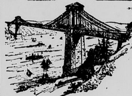
NEW HUDSON RIVER BRIDGE.
