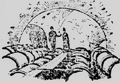
OUTLET FROM RESERVOIR.
